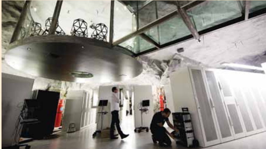
A man walks inside the Pionen White Mountains high-security computer storage facility of Swedish Internet service provider Bahnhof in Stockholm. The Pionen data center, once a Cold War era nuclear bunker, is one of the most well-protected in the world.
