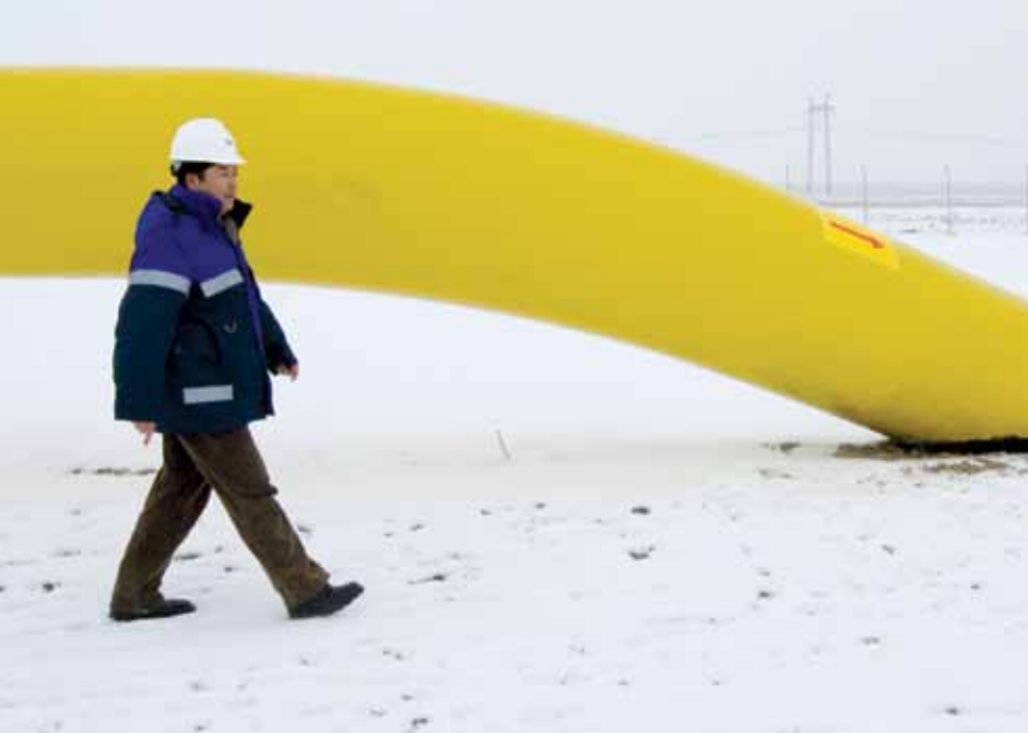
The gas pipeline that begins in Turkmenistan and transits Uzbekistan and Kazakhstan on the way to China is an example of multilateral cooperation in Central Asia.
