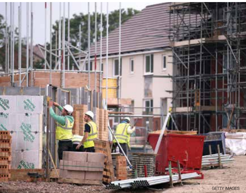
Construction workers build new houses in Bristol, England. The British construction industry provided plentiful employment for immigrants from Eastern Europe.
