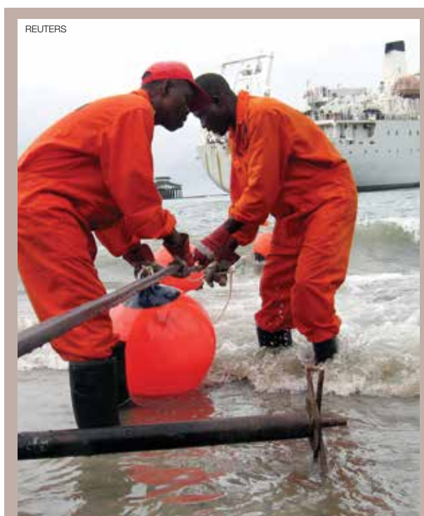
Workers lay fiber optic cables near the coastal city of Mombasa, Kenya, in June 2009. Eleven undersea fiber-optic cables have been laid in Africa in the last few years, providing faster and more affordable Internet connections.
