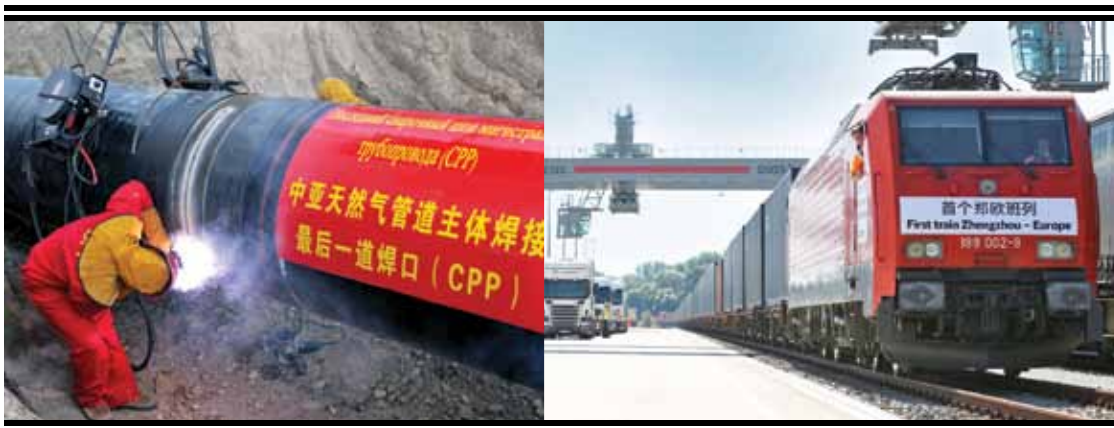
Workers weld the last links of Kazakhstan's segment of the Central Asia-China gas pipeline near Almaty in 2009.
