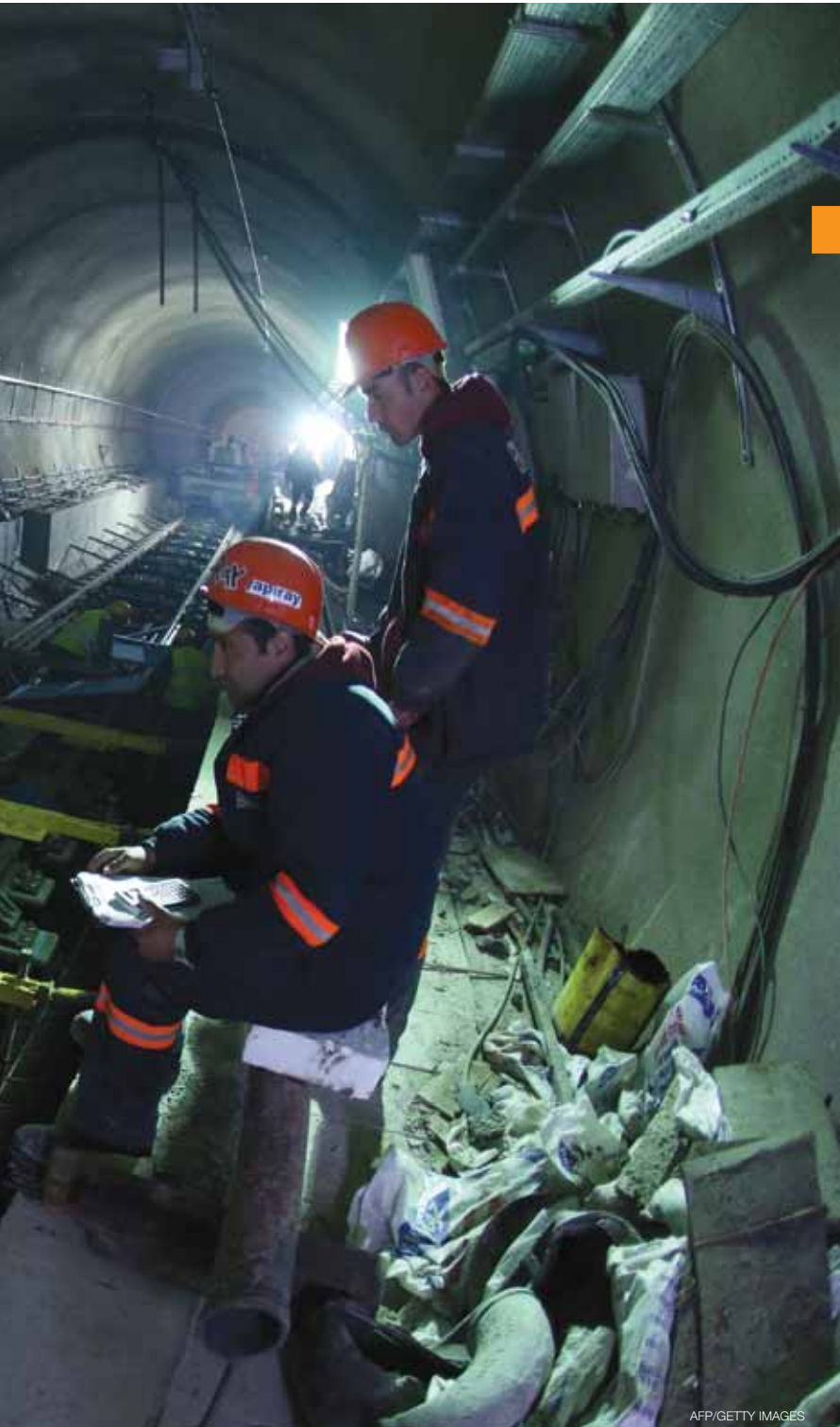
Turkish workers build a railway in the Marmaray Tunnel under the Bosphorus Strait in April 2013. The Marmaray project, which reflects Turkey's new economic confidence, includes the undersea tunnel and the modernization of suburban rail lines along the Sea of Marmara.
